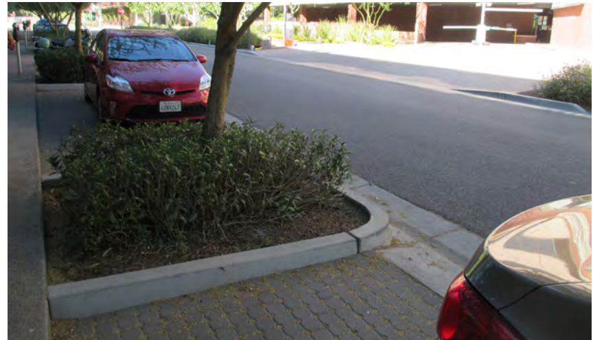
Grated curb cuts convey stormwater from pavement into planting areas.
