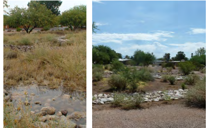
Bioretention areas detain stormwater while enhancing the landscape.
