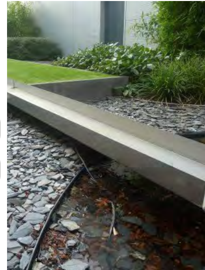
Disconnecting a downspout allows rainwater to supplement irrigation in the landscapes.
