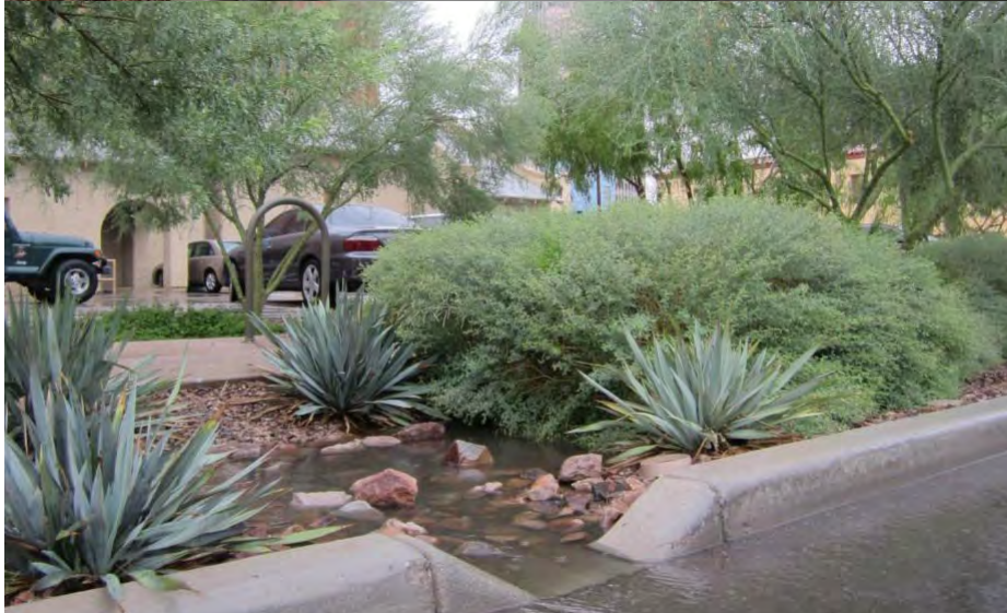
Curb cuts at the street edge capture significant flows during rainfall events.
