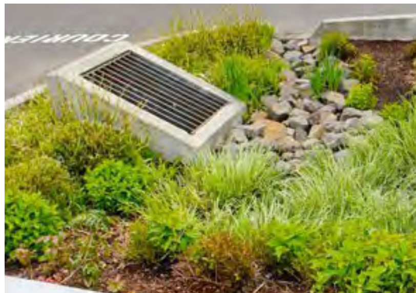
A Bioretention Cell with sloped grate and sediment capture in landscaped area
