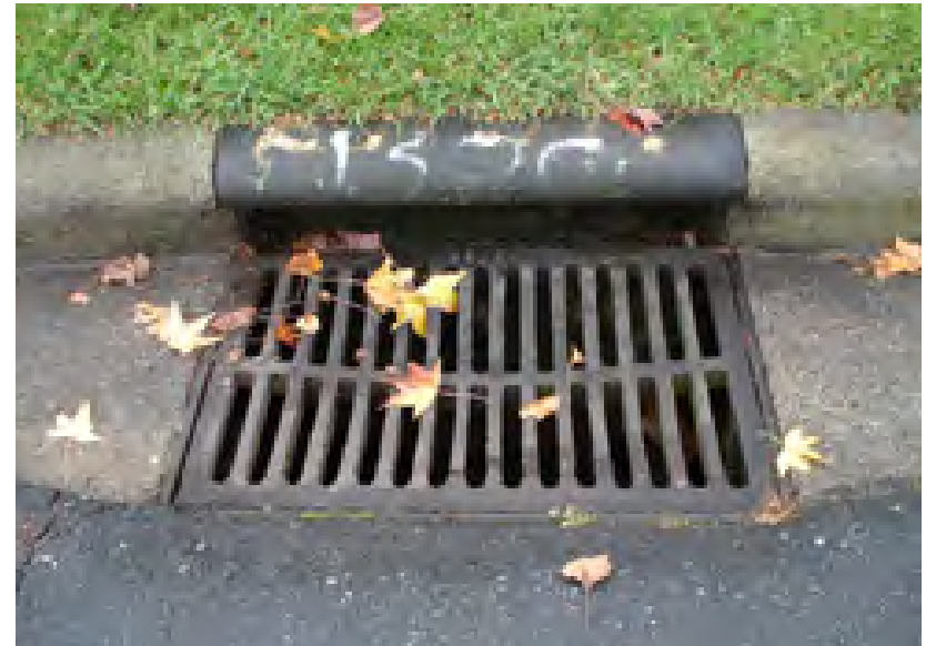
Catch Basins have been used for centuries to capture surface water and convey it into underground pipes.
