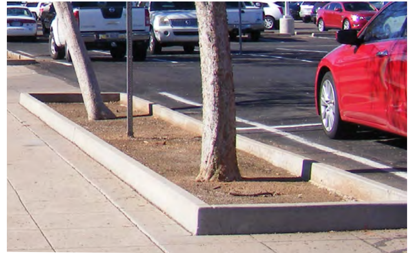
The growth potential and lifespan of trees can be restricted by standard tree planters due to impervious surfaces and compacted subgrades.
