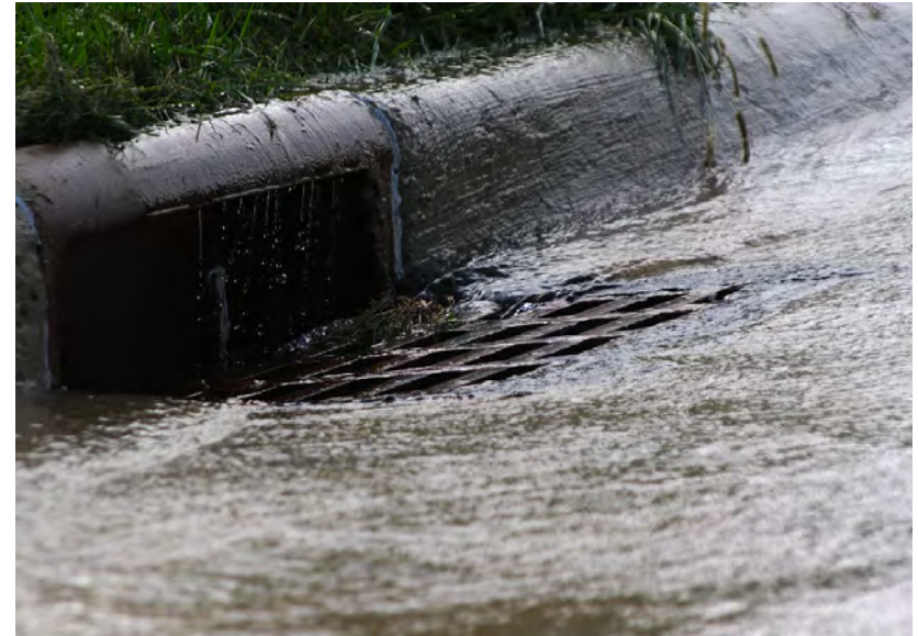
Existing Standard Curbs keep stormwater out of landscaped areas.
