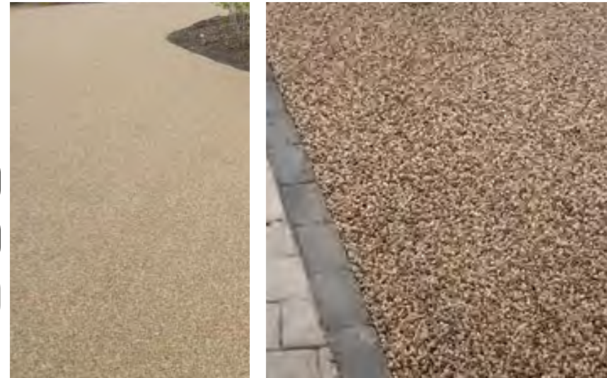
Stabilized aggregate reduces storm runoff from paved low-traffic areas.
