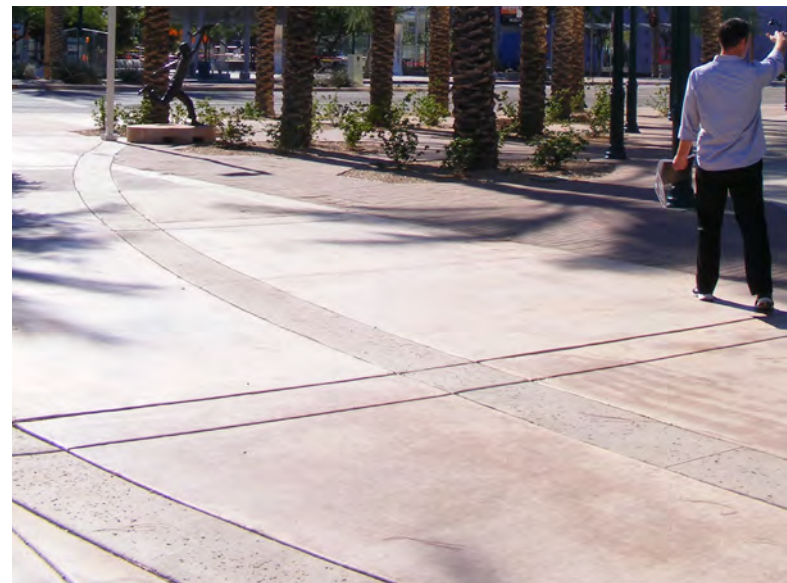
Impervious pavements are typical in urbanized areas, but result in increased volume and velocity of stormwater runoff, affecting downstream hydrology.
