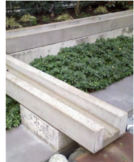
Disconnecting a downspout allows rainwater to supplement irrigation in the landscapes.
