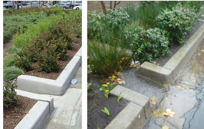
Curb cuts direct stormwater from street to landscape areas.
