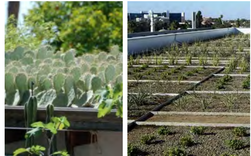
Green roofs store and utilize stormwater to reduce runoff from building sites.
