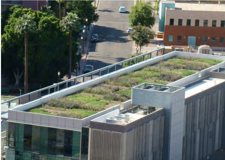
Green roofs absorb rainwater, provide insulation and create wildlife habitat. It also helps to lower adjacent air temperature, mitigating the heat island effect.
