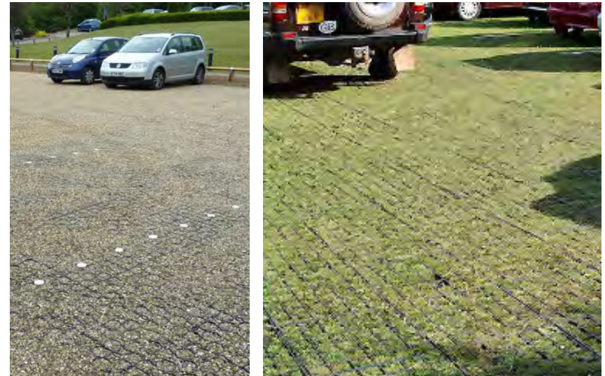
Structural grid paving reduces runoff in parking areas and firelanes.
