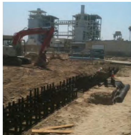
Silva Cell tree structures used for LID purposes in Burbank, CA (courtesy Silva Cell Products).
