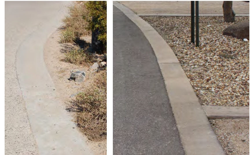
Flush curbs allow stormwater to sheet drain to landscape areas.
