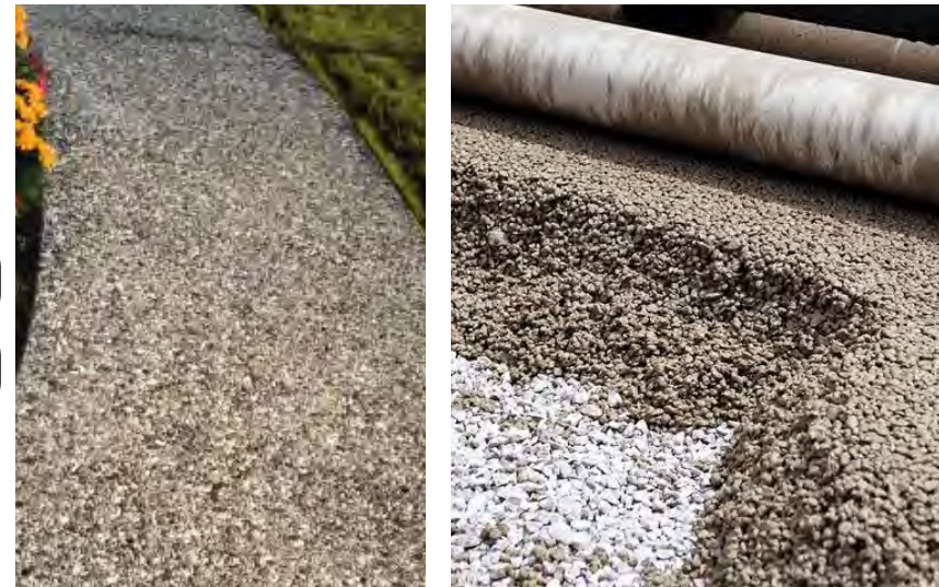
Porous concrete can reduce runoff in sidewalks and plaza areas.
