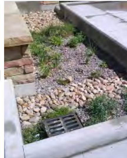
Bioretention cells fit into constrained urban site.
