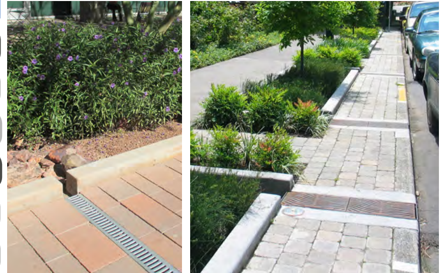
Grates allow stormwater to pass through while proving an accessible pedestrian route.
