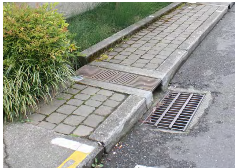
A Grated Curb Cut conveys stormwater across a sidewalk
