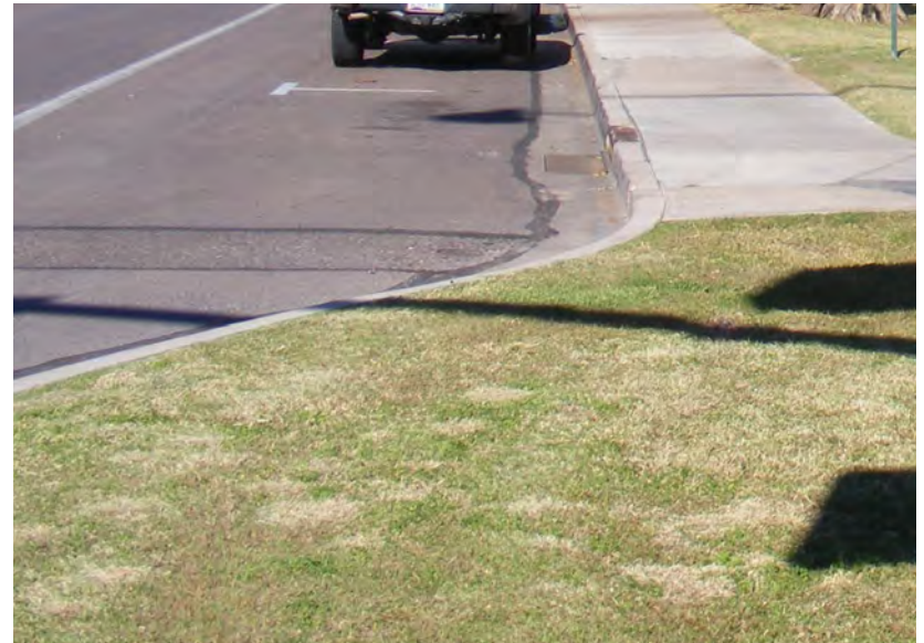
Existing standard curb and gutter conveys stormwater to a piped system underground.
