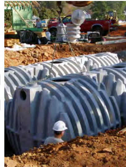
Underground cisterns provide storage areas for rainwater reuse.
