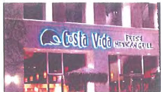
Example of internally illuminated reverse pan-channel letters.
