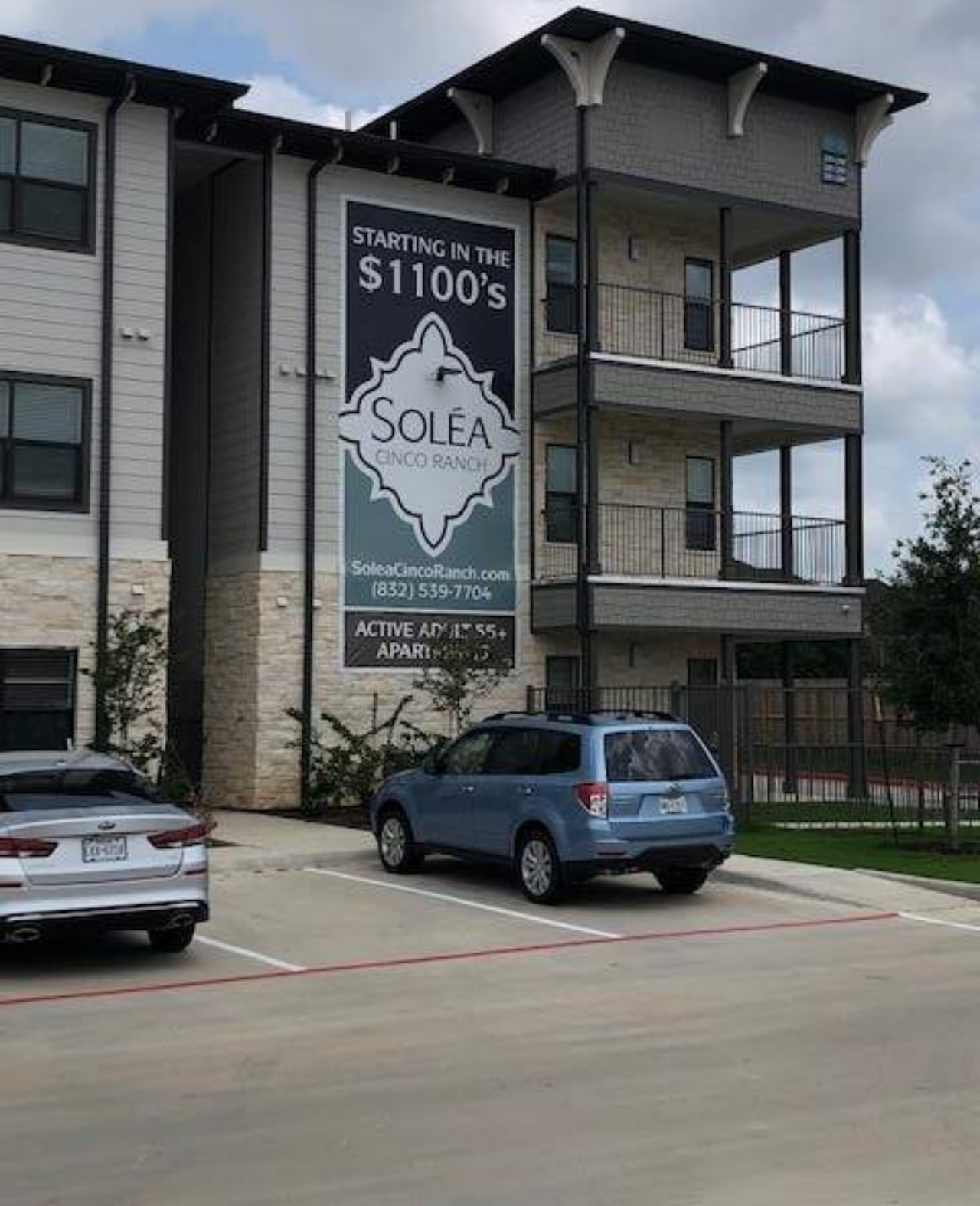
Temporary Wall Sign Example
